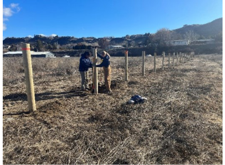
Fence installation by Washington Conservation Corps members
