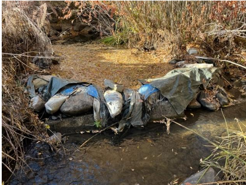
Figure 3. Looking upstream at diversion
